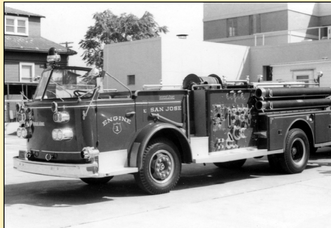
Left: This is the way San Jose Fire Department's Engine 1 looked when it was in service at 201 N. Market Street. The 1958 American LaFrance Series 900 pumper had a 500-gallon water tank and was capable of putting out 1,250 gpm.
